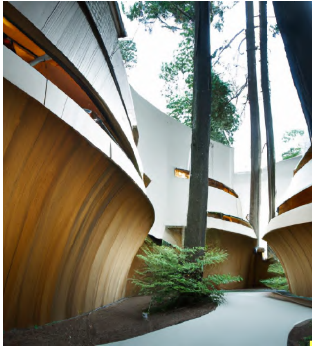
Architecture, buildings, wings
